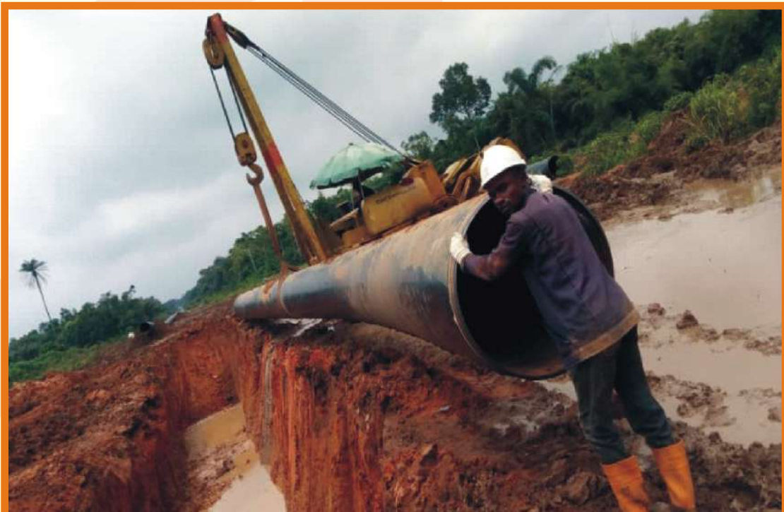
Construction of 36" x 20km Dangote Refinery & Fertiliser Gas Pipeline
