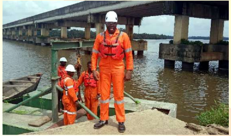
CEO AT SAVANNAH PROJECT SITES CALABAR
