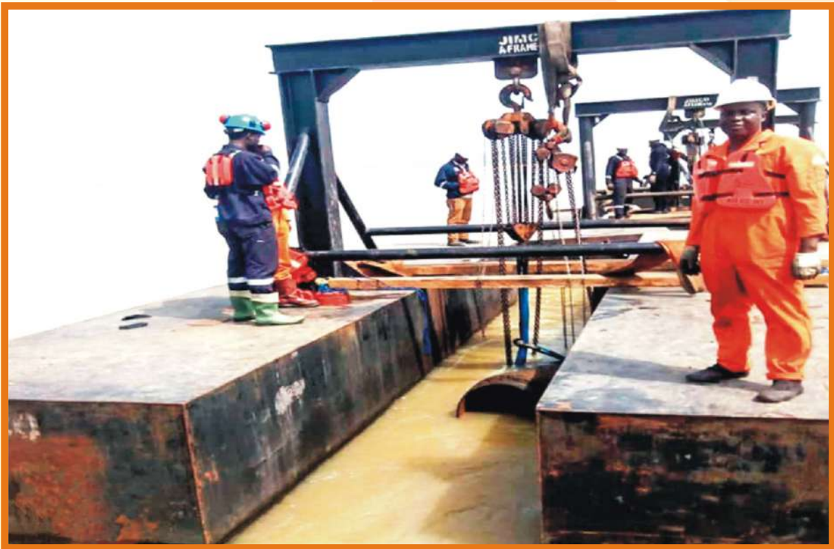
24" x 1.3km River Niger Agip Kwale-Akri Gas Pipeline Repair
