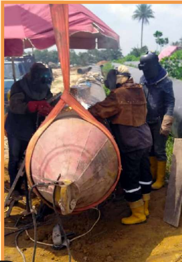
18" x 1.2km Egbema Power Gas Pipeline PIPELINE CONSTRUCTION
