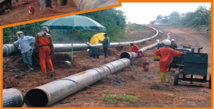
18" x 1.2km Egbema Power Gas Pipeline PIPELINE CONSTRUCTION
