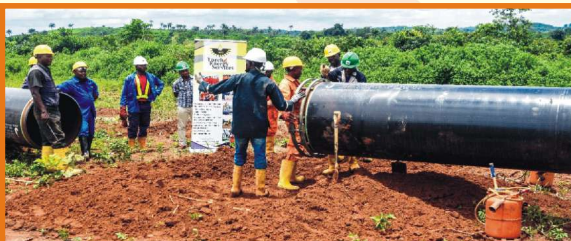
Construction of 36" x 20km Dangote Refinery & Fertiliser Gas Pipeline
