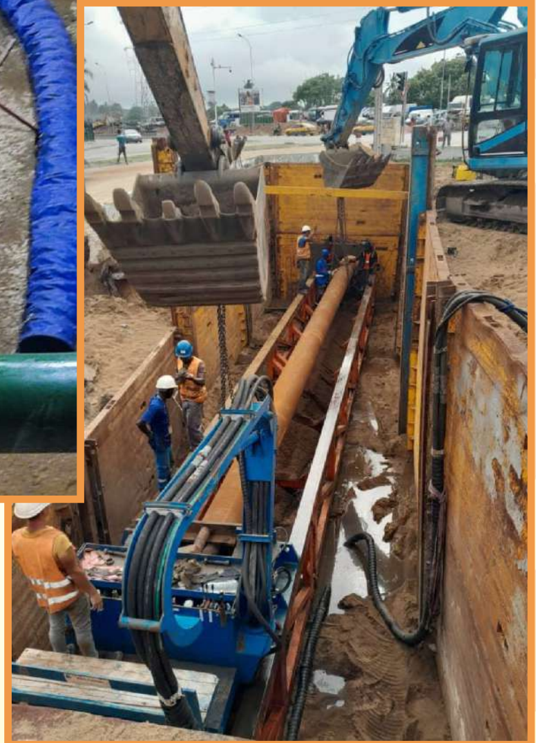
Welding completion at KP 00
