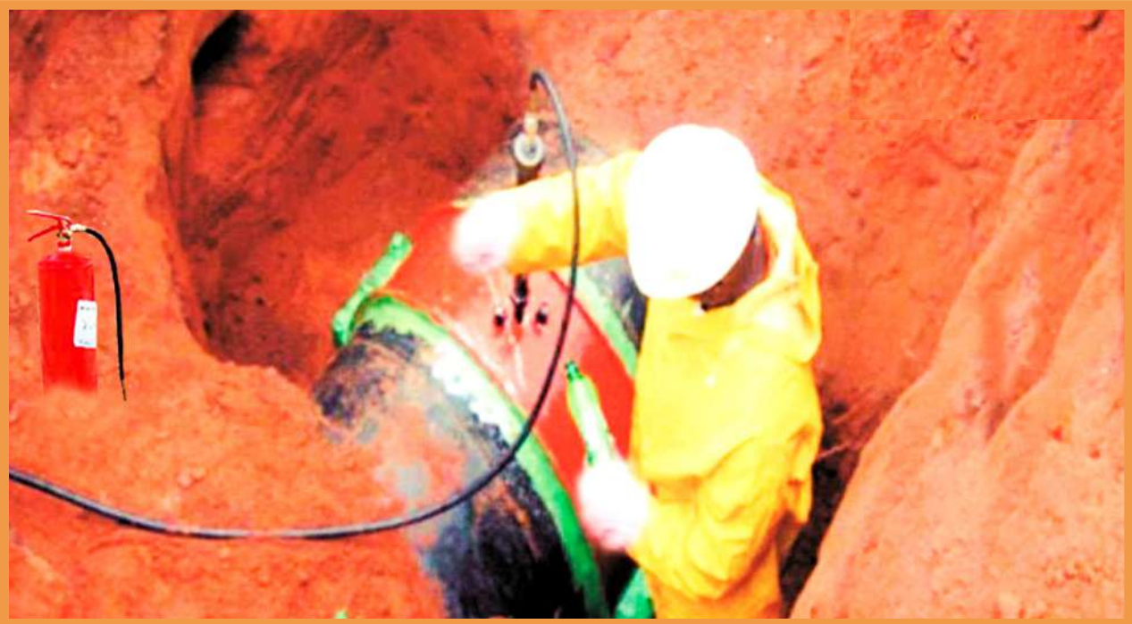
On-line Pipeline Leak repair on 30" Ughelli Gas Pipeline
