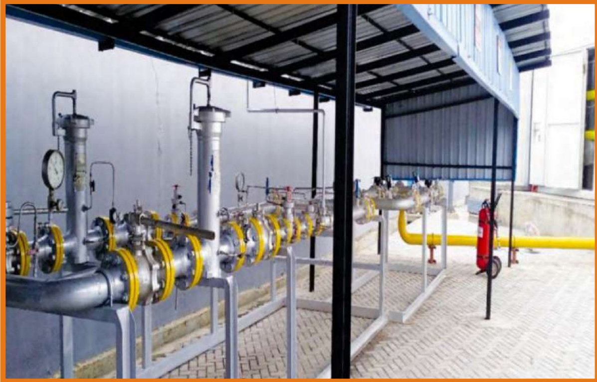
FABRICATION AND INSTALLATION OF 9.0 MMSCFD AT GASCO MARINE ABEOKUTA
