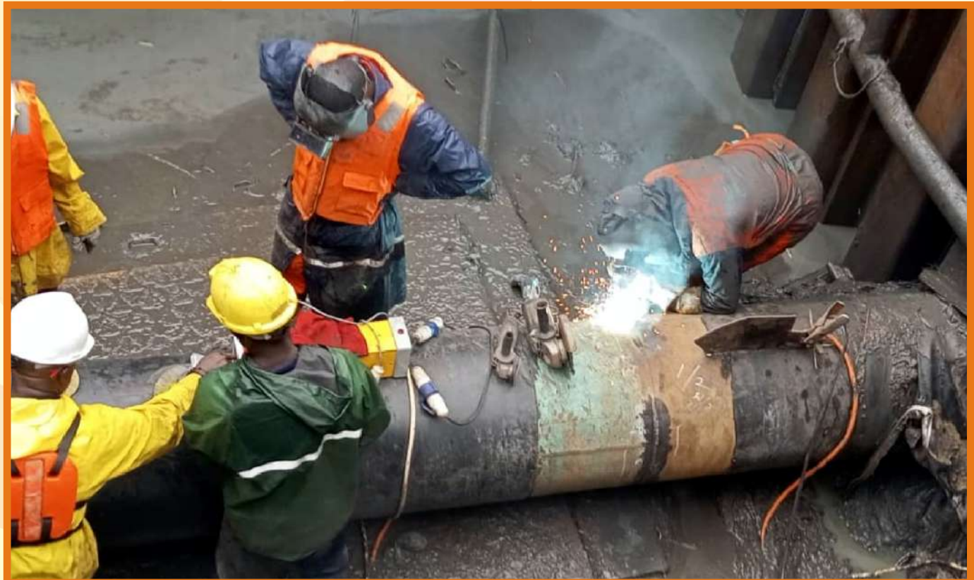
24 Inches Oron Gas Pipeline Repair Project (SWAMP)
